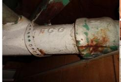
6- A sizable crack was discovered on the verticle drain pipe located in the basement ceiling. Have a plumber review and correct as needed.
