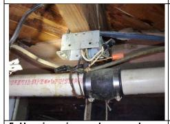
5- Hanging wires and exposed splices were discovered in the crawlspace sealing at three locations. Have a licensed electrician review all wiring in the crawlspace and effect corrections so that industry safe wiring practices will exist
