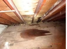
7- Active water leakage was observed in the attic area located above the garage. Have a roofer review and correct so that no further leaking will occur. The leaks appear to be generated from a satellite dish attached to the roof surface in this location.
