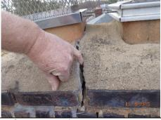
4- Consult a chimney mason to review the chase that serves the fireplace, the furnace and the water heater. Excessive cracking is present at the chimney's crown. Allow for extensive repairs!
