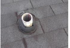
3- The rubber boots around vent pipe seals are in a depleted state and need attention from a roofer.
